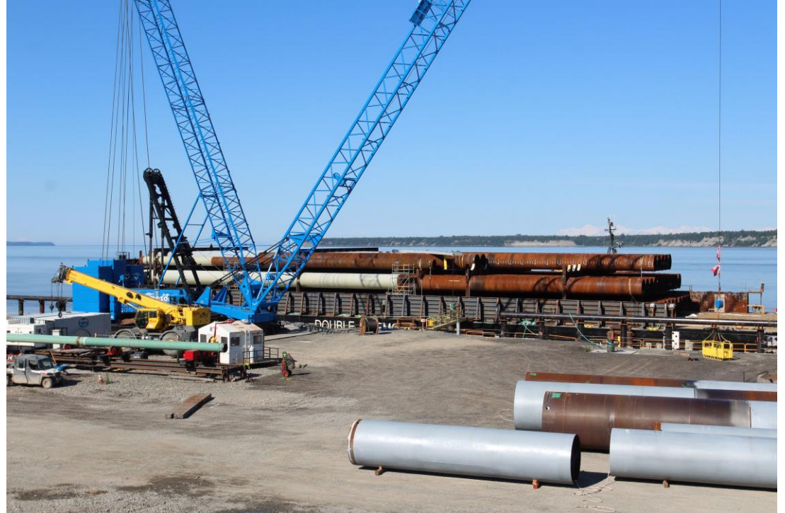
Pile barge being unloaded at the berthing facility.
