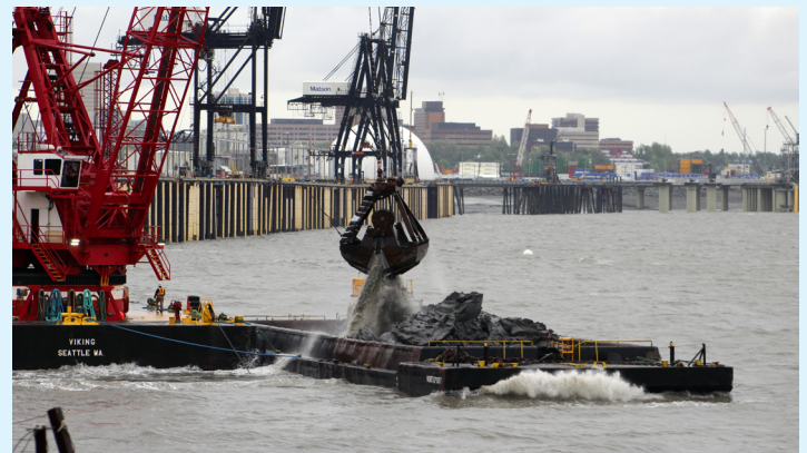
NES1 marine-based dredging widens the shipping canal making it safer for vessels to dock at the Cargo Terminals.
