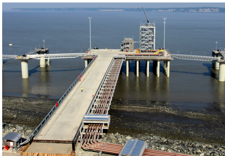
The new Petroleum and Cement Terminal.
