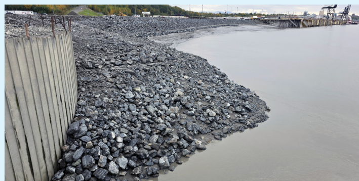
View of completed NES1.
