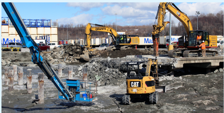
Trestle 1B demolition.
