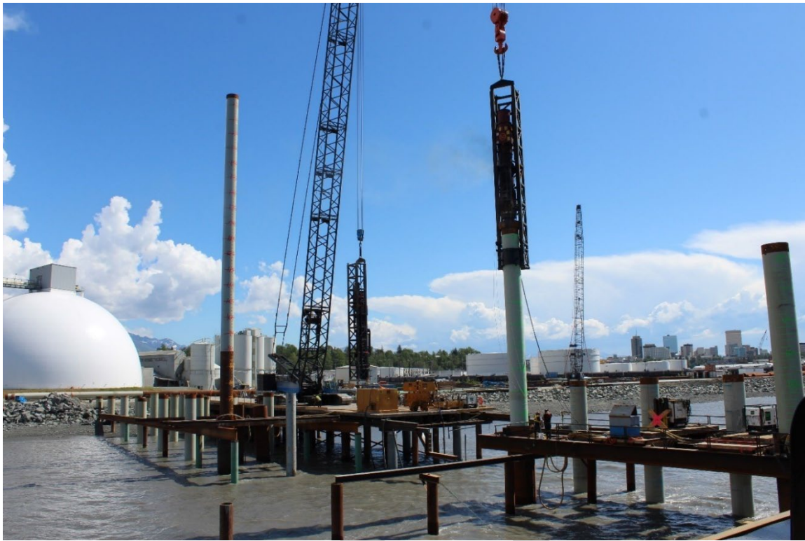
Figure 4-19. Typical Temporary Work Platform, Petroleum and Cement Terminal, Port of Alaska
