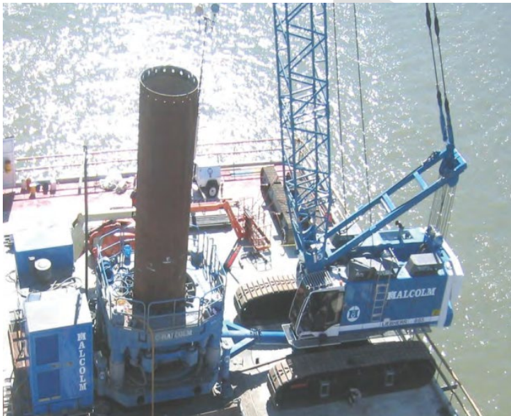
Figure 5-16. Oscillator Equipment for Drilled Shaft Construction, Far (Source: FHWA 2010)
