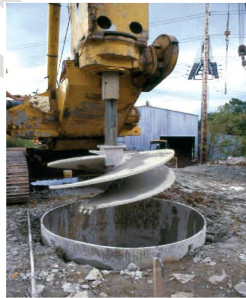
Figure 5-17. Auger Equipment for Drilled Shaft Construction, Close (Source: FHWA 2010)
