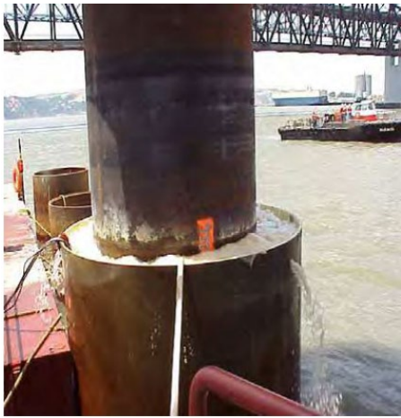
Figure 5-2. Confined System at the Benicia-Martinez Bridge (Source: Caltrans 2015)
