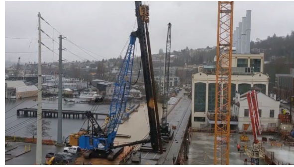
Figure 5-19. Helical Pile Installation System (Crane, Driver, and Guide) (Source: Included with permission from Pileworks)
