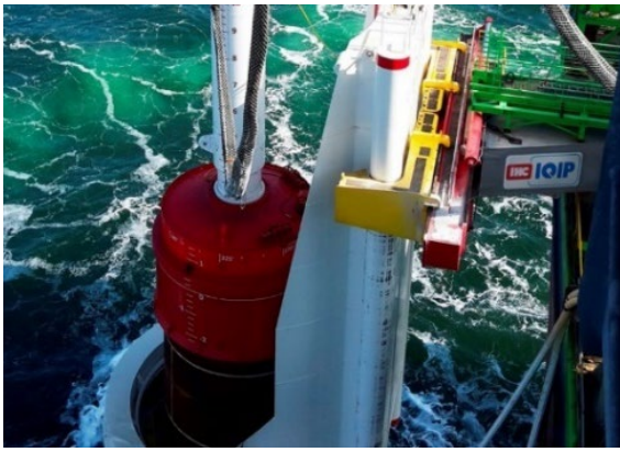
Figure 5-12. Integrated Monopile Installer, Close (Source: Included with permission from IQIP 2022b)
